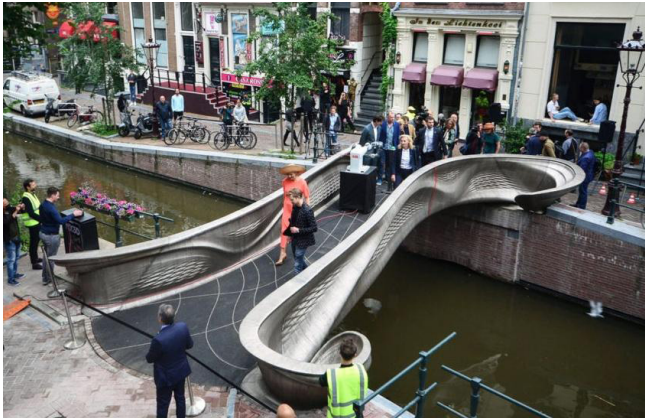
Figure 4. 3D-Printed Stainless-Steel Bridge in Amsterdam 45
